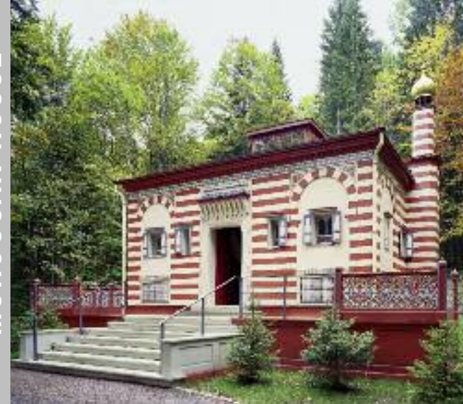
Moroccan House (top); Central hall of the Moroccan House (bottom)
